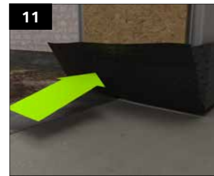
Where apertures are found at ground level fold up the excess DPC and temporarily fix in place, this can be done with tape or other method.
