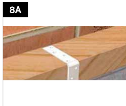
The Galvanised wall straps - 30mm wide by 2.5mm and 1m long (not supplied by Ultraframe).
