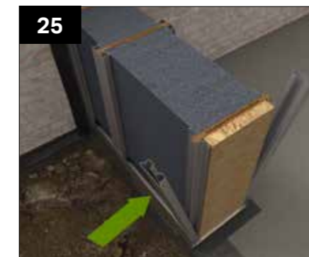
Fit the walling panel and aperture panel together using the steel full clips, using the same method as previously used for attaching walling panels together. Please note:- for Tiled Roof & Flat Roof the clips will extend beyond the tops of the walling panels and internal and external clips will differ in length.
