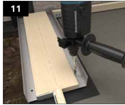
Through the punched holes in the base trays pre-drill the foundations using appropriate size drill bit for fixings (not supplied). Example fixing: M6 x 85mm Concrete Bolt with a 1kN pull out @ 600mm max centres or similar suitable approved for the substrate. Refer to fixing table at start of guide.
