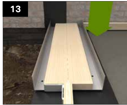
Fix the trays down to the basework using appropriate fixings (NOT SUPPLIED) through pre punched holes. M6 x 85mm Concrete Bolt with a 1kN pull out @ 600mm max centres or similar suitable approved for the substrate. Refer to fixing table at start of guide.
