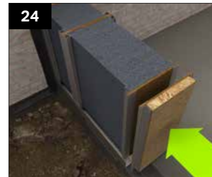
When an opening in the wall is reached, an aperture panel is used to terminate and allow for secure window fixing. Locate the relevant aperture panel and position this against a walling panel, as shown on the location plan.
