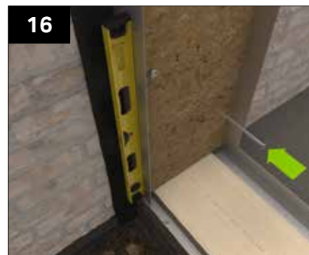
Ensuring the host wall tray is plumb and level secure it into the host wall using appropriate fixings (NOT SUPPLIED). Example fixing: Concrete Frame Screw 7.5x70mm this may require pre-drilling at staggered 300mm centres or other similar approved fixing for the substrate, avoiding mortar joints. Refer to fixing table at start of guide.
